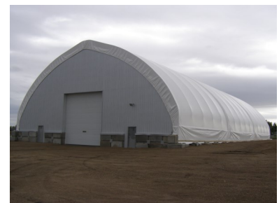
Freestanding 80' Welded Truss
