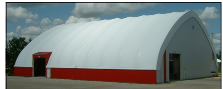
Freestanding 110' Welded Truss
