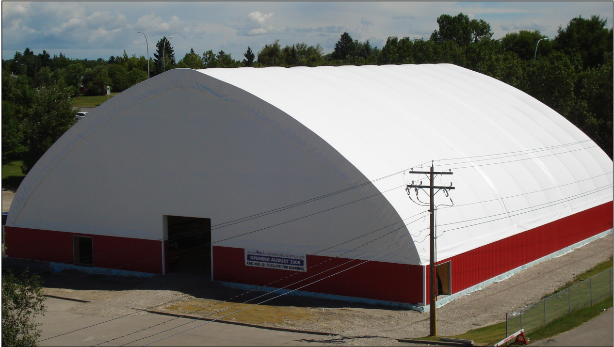
Freestanding 120' x 132' Welded Truss Baseball Practice Academy
